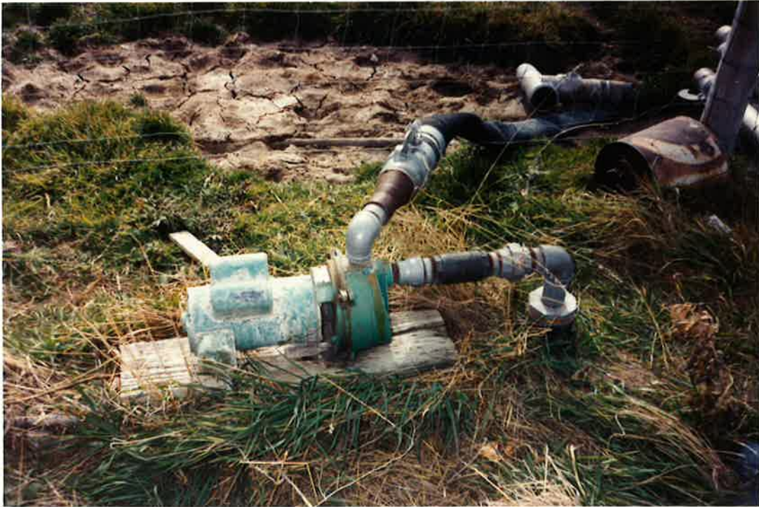
* Diverting Works (facing South)
