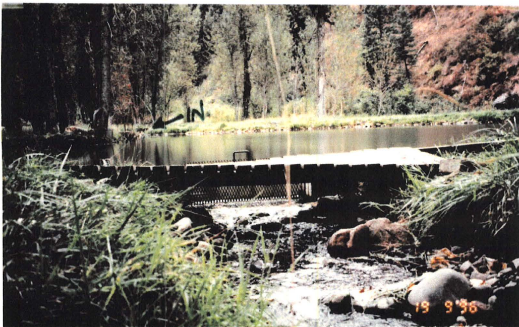
Pond outlet Meas. taken in current Structure w/ Screen removed. Inlet on opposite side
