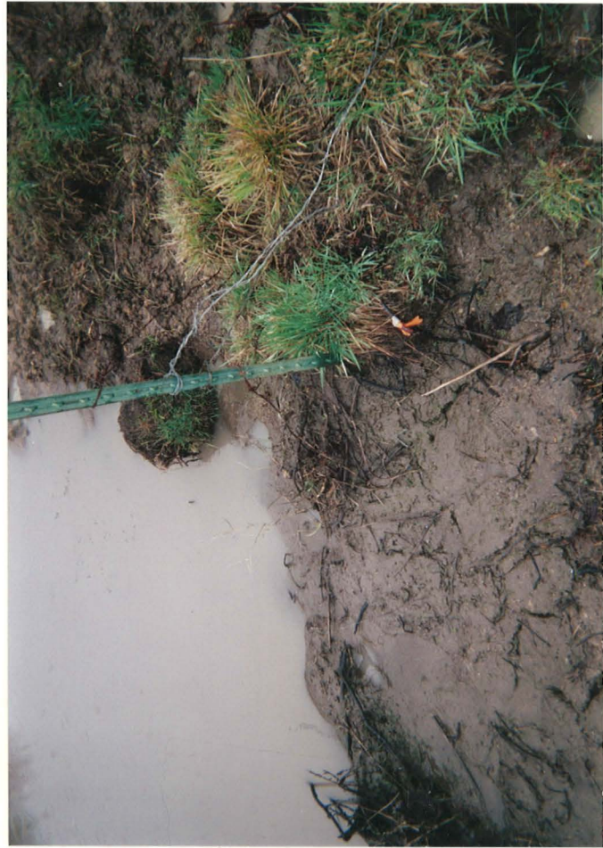
Tarter Claim Joselin Ditch Pipe #2 Inlet
