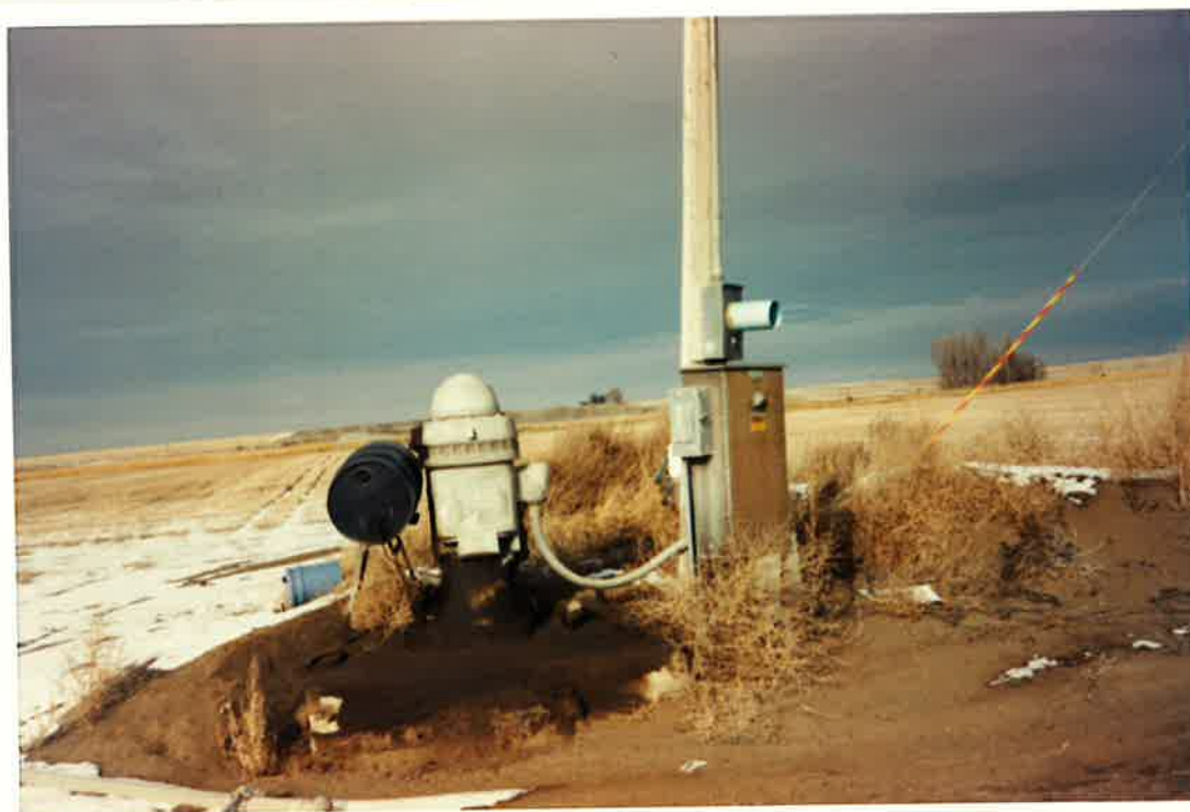
* Point of diversion (Facing North)
