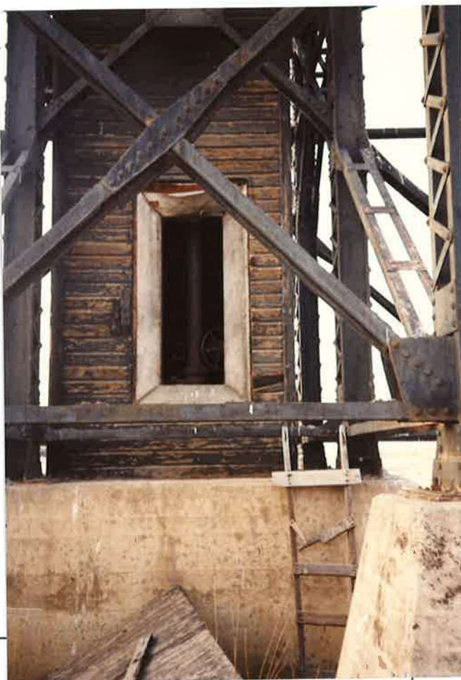
Kimama Union Pacific water tower, close up of opening to piping.
