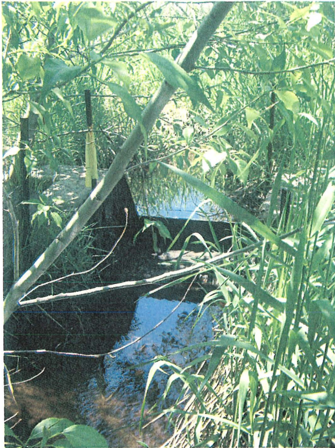
Photo of Ridenour weir from just downstream. POD off Rush Creek is about 100 yards upstream of this point.
