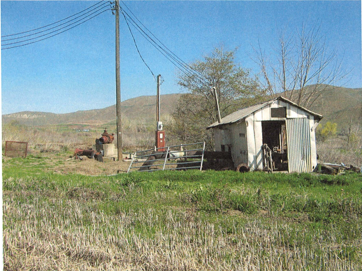
POD. Picture taken by Monica Van Bussum. This shows POD for systems 3 and 4.
