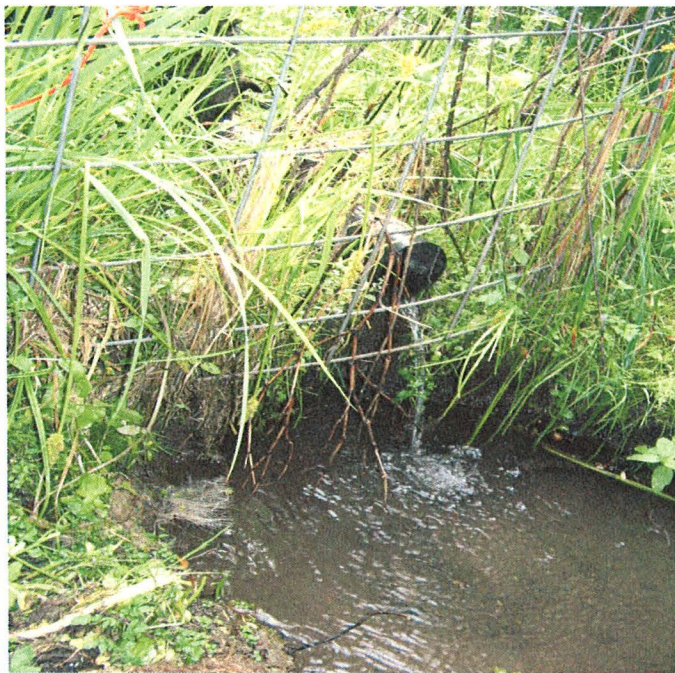
View of overflow pipe from spring / water not used for irrigation.
