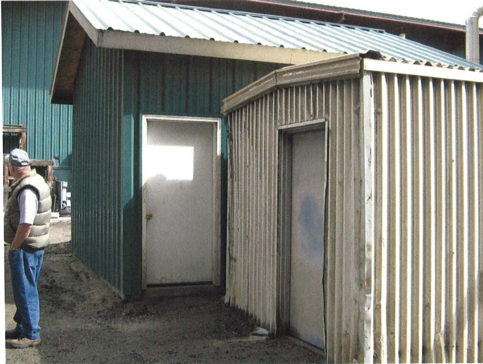
Buildings housing the wells. The green (north) building houses the 2001 well and the white building houses the 1982 well.
