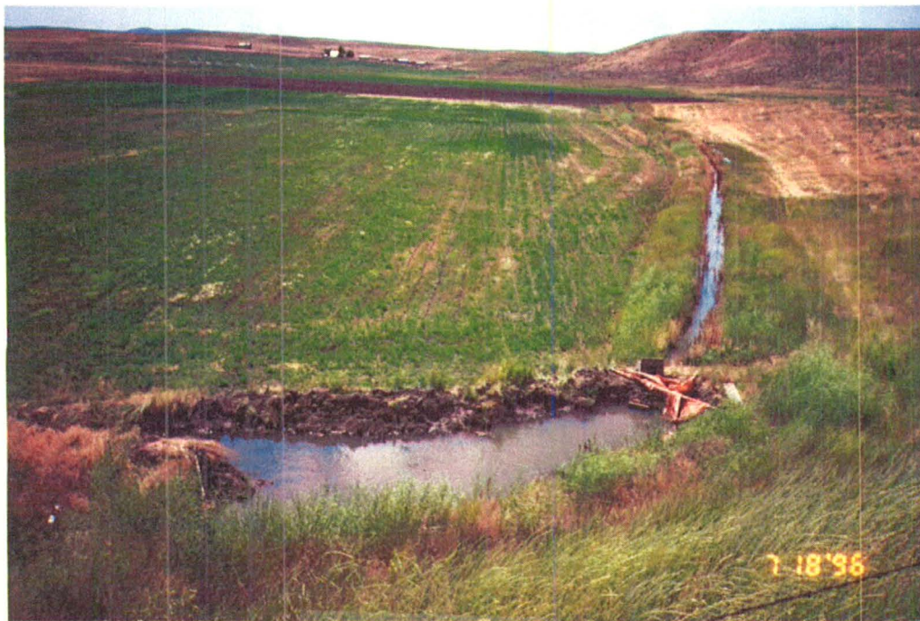
P/u looking west from dam. Res. outlet is submerged in pool below. Ditch to right serves upper fields
