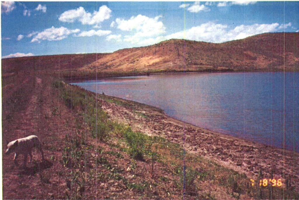
Dam SENE Sec 26 view to North
