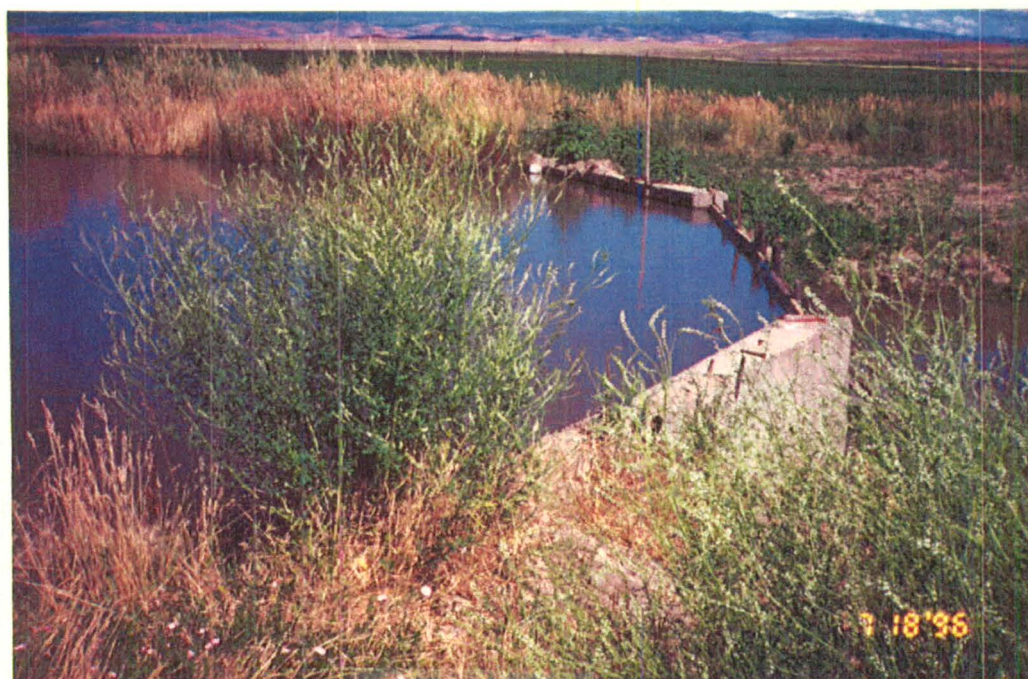
Check dam & pool in Hog Creek.
