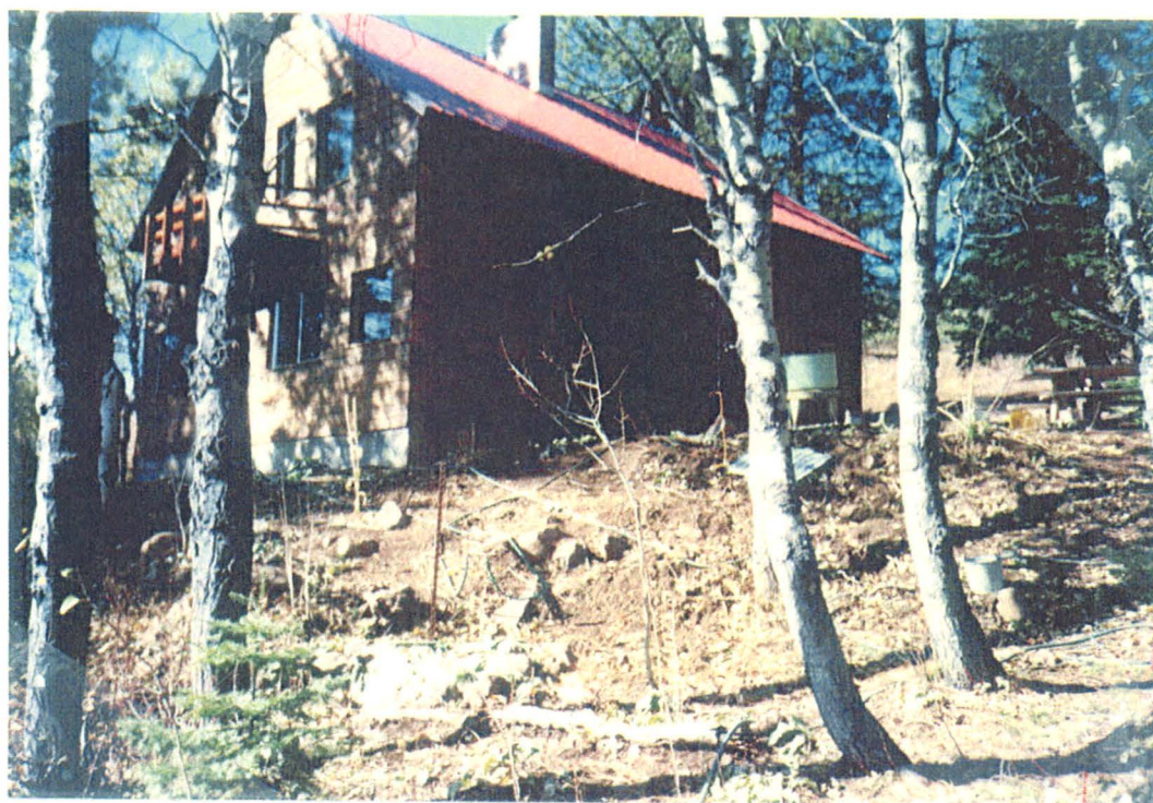
P.D. Cabin pipes & boxes are visible in lower center of photo. Looking Northwest.
