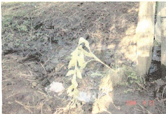
Soil Erosion around trough
