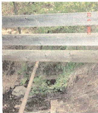
Pipeline to FS trough from cistern.
