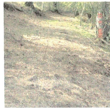
Access Road and buried pipeline
