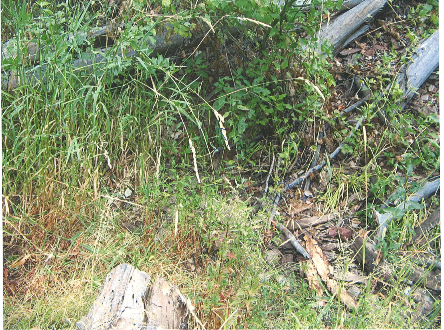
67-4549 View of ditch just below spring source. Needs repair after high water year and poor health of claimants.
