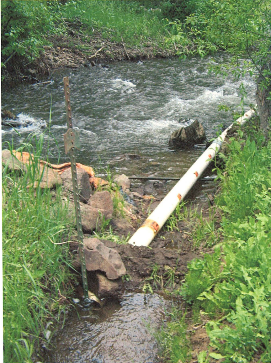
A0017648. Normally a 12" pipe is in place. The claimants were not irrigating yet and so had a smaller pipe in the ditch for stock.
