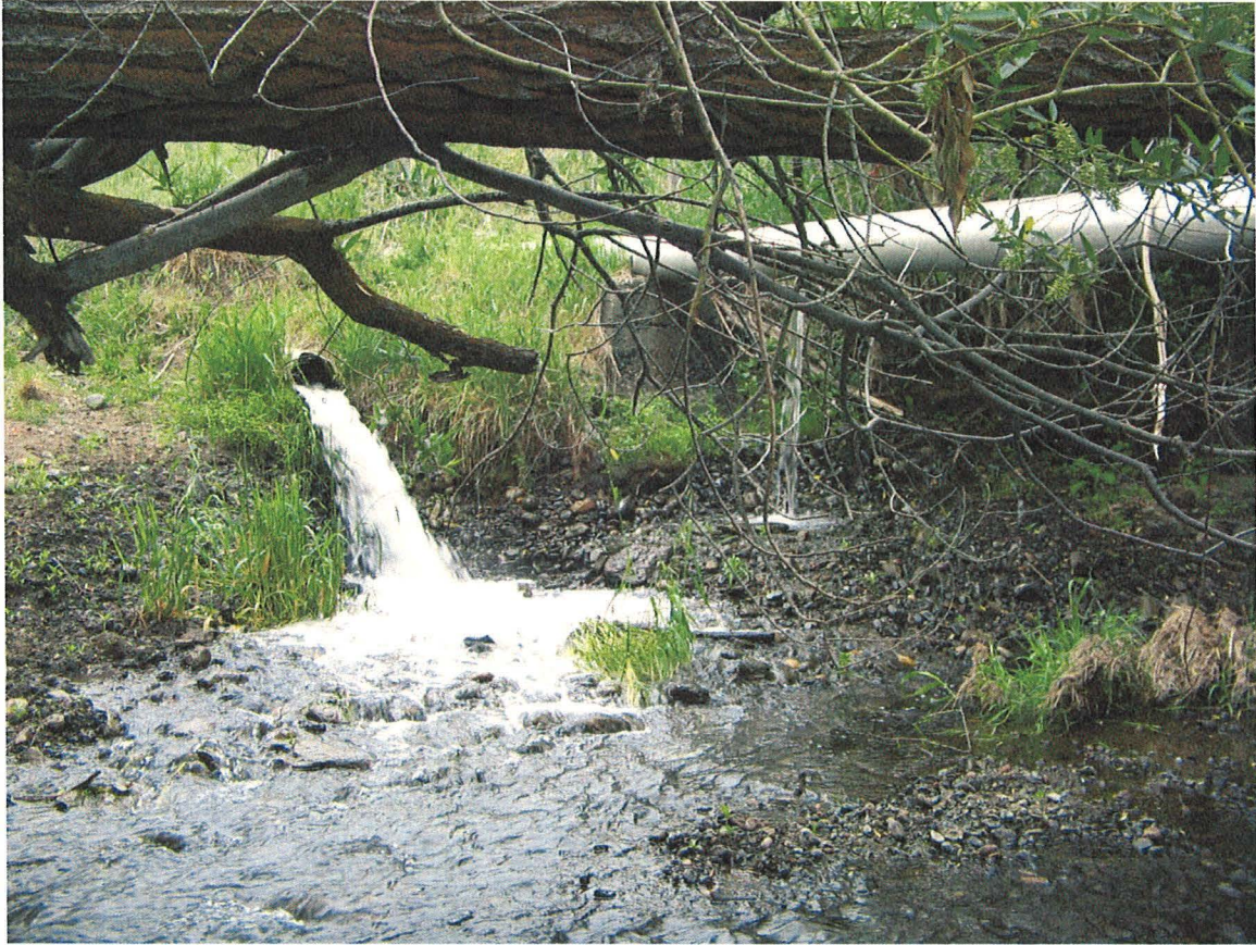
The pipe shown spilling into Banner Creek here is Middle Valley Ditch water. Bonner uses very little of this water, although he owns a number of shares. He is using Banner Creek water almost exclusively, as opposed to Middle Valley Ditch water. Photo taken facing north-northeast.
