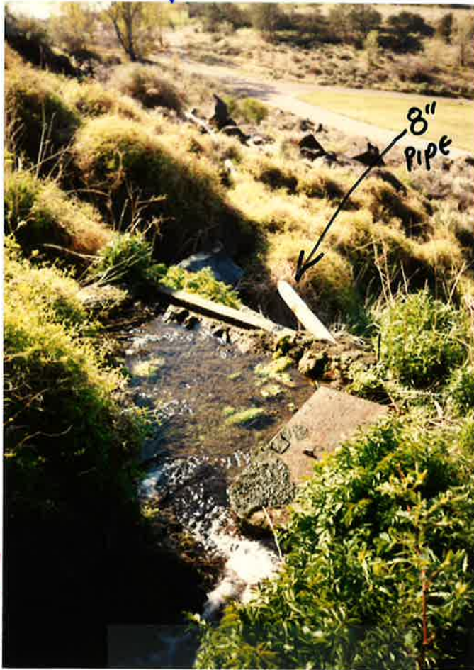
DIVERSION WITH 8" PIPELINE @ NIAGARA SPRINGS.
