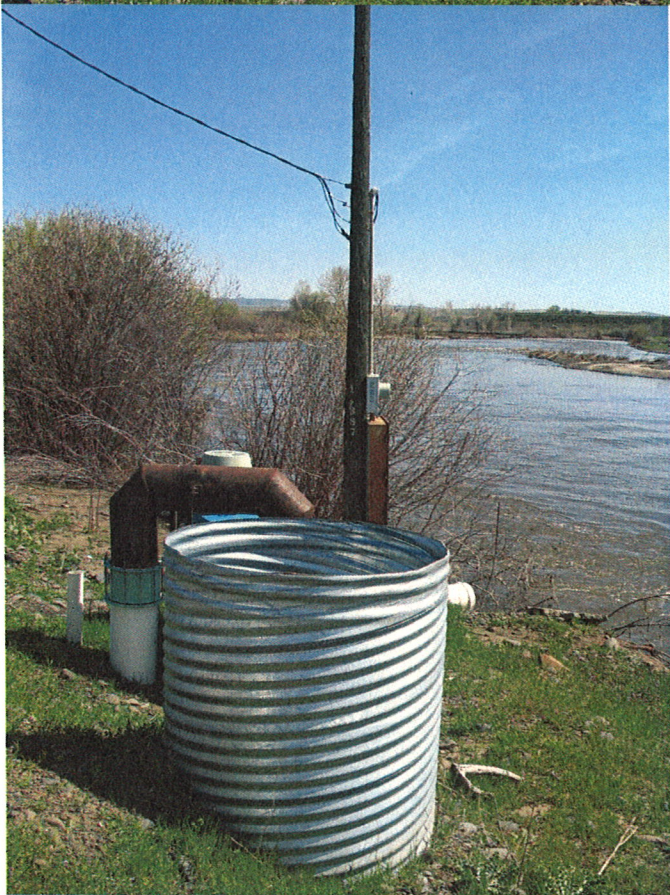
A0017628. 67-4150. Scarrow pump off the Weiser. First picture is taken looking upstream. Second picture is looking downstream.
