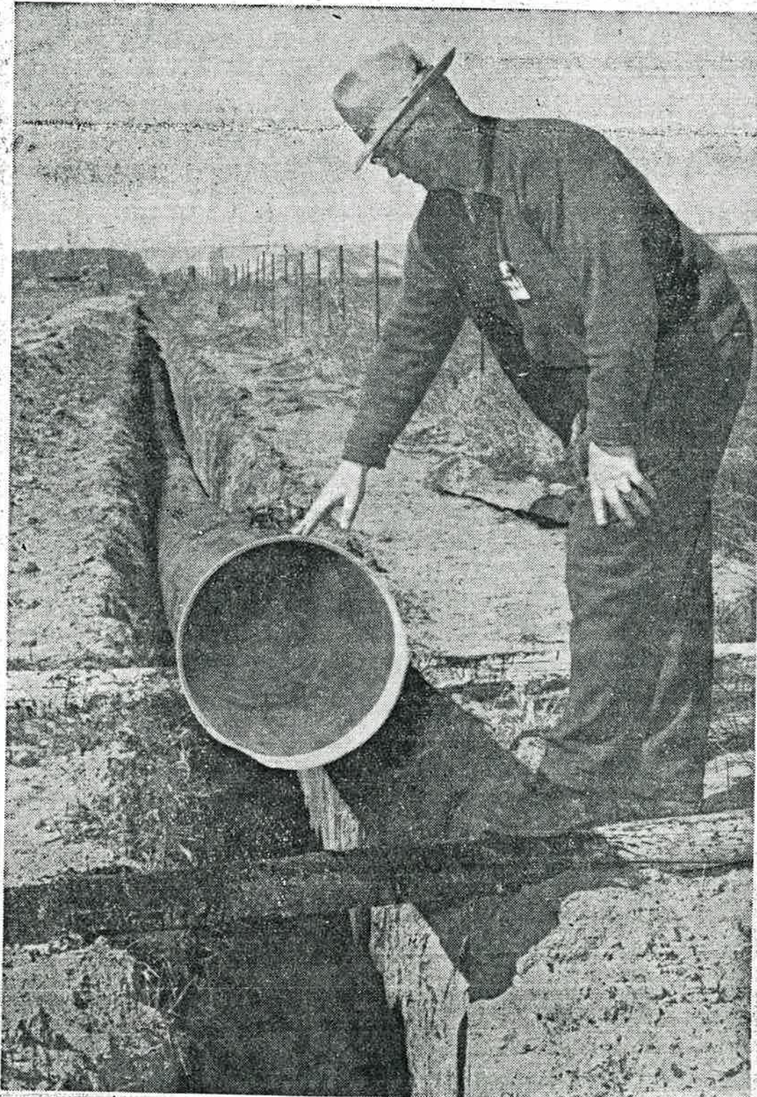
Emerson Pugmire, mayor of Hagerman, points to the end of the new water main addition. The new addition is 9,000 feet long and is made entirely of four-foot incendiary bomb casings. (Staff photo-engraving)
