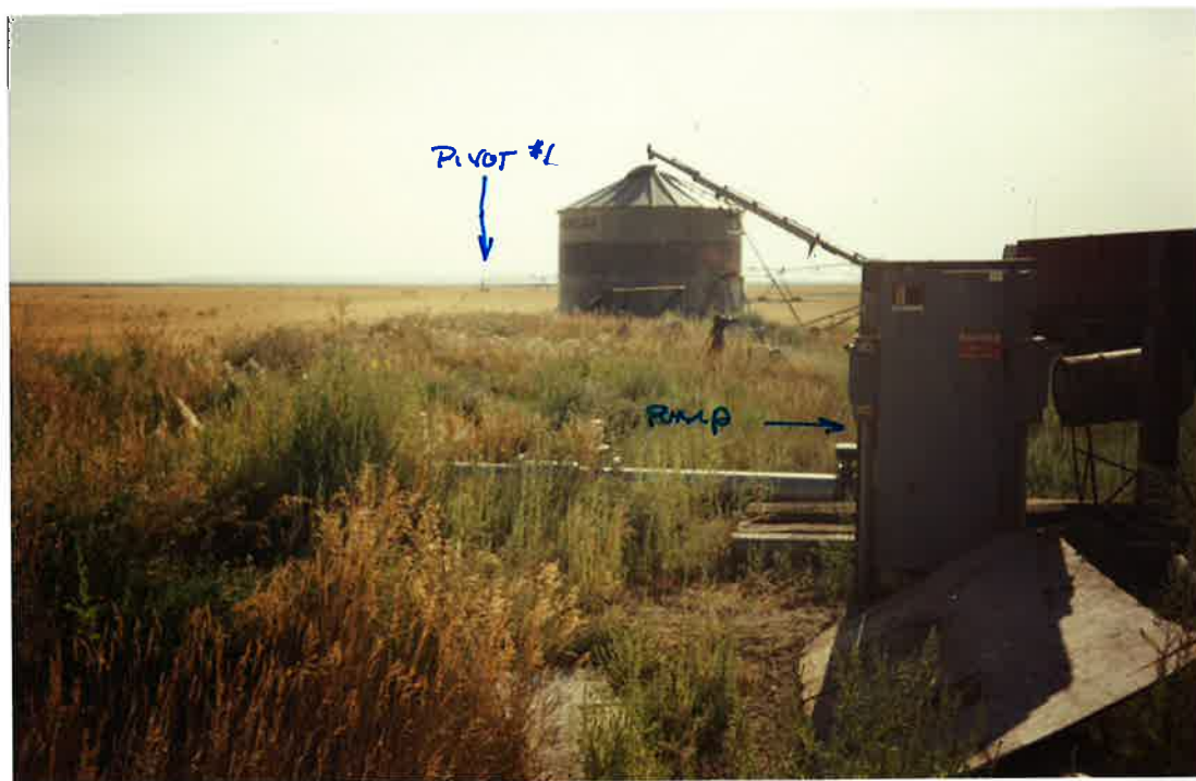
Photo # 1-11 LOOKING EAST FROM THE POD SHOWING THE PUMP ELECTRICAL JUNCTION BOX WITH PIVOT # 1 IN THE BACKGROUND TO THE EAST.
