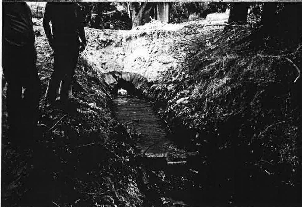
1' contracted rectangular weir meas. total output from spring, when pump turned on pump easily adjusted to consume total flow. During exam pump started and outflow ceased to flow.
