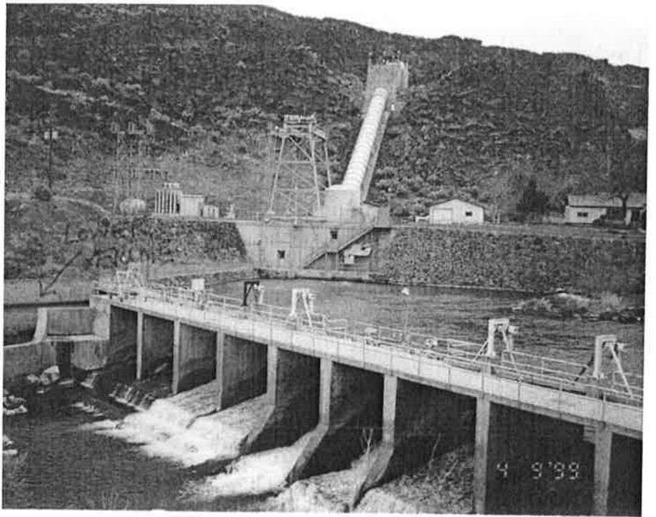
Upper Malad Plant, discharge pool, diversion to lower flume & spill to river
