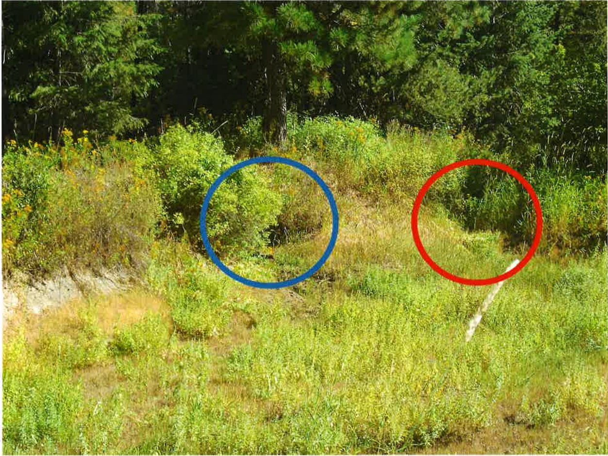
Figure 5- Point where creek drains into dugout/pond that does not hold water (blue circle, left). Point where water drains out of dugout/pond heading east, then turning south (red circle, right).
