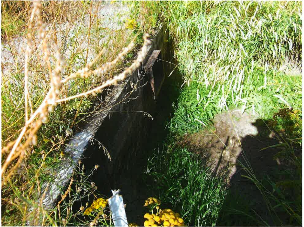
Figure 3- Original culvert for creek to run under path.
