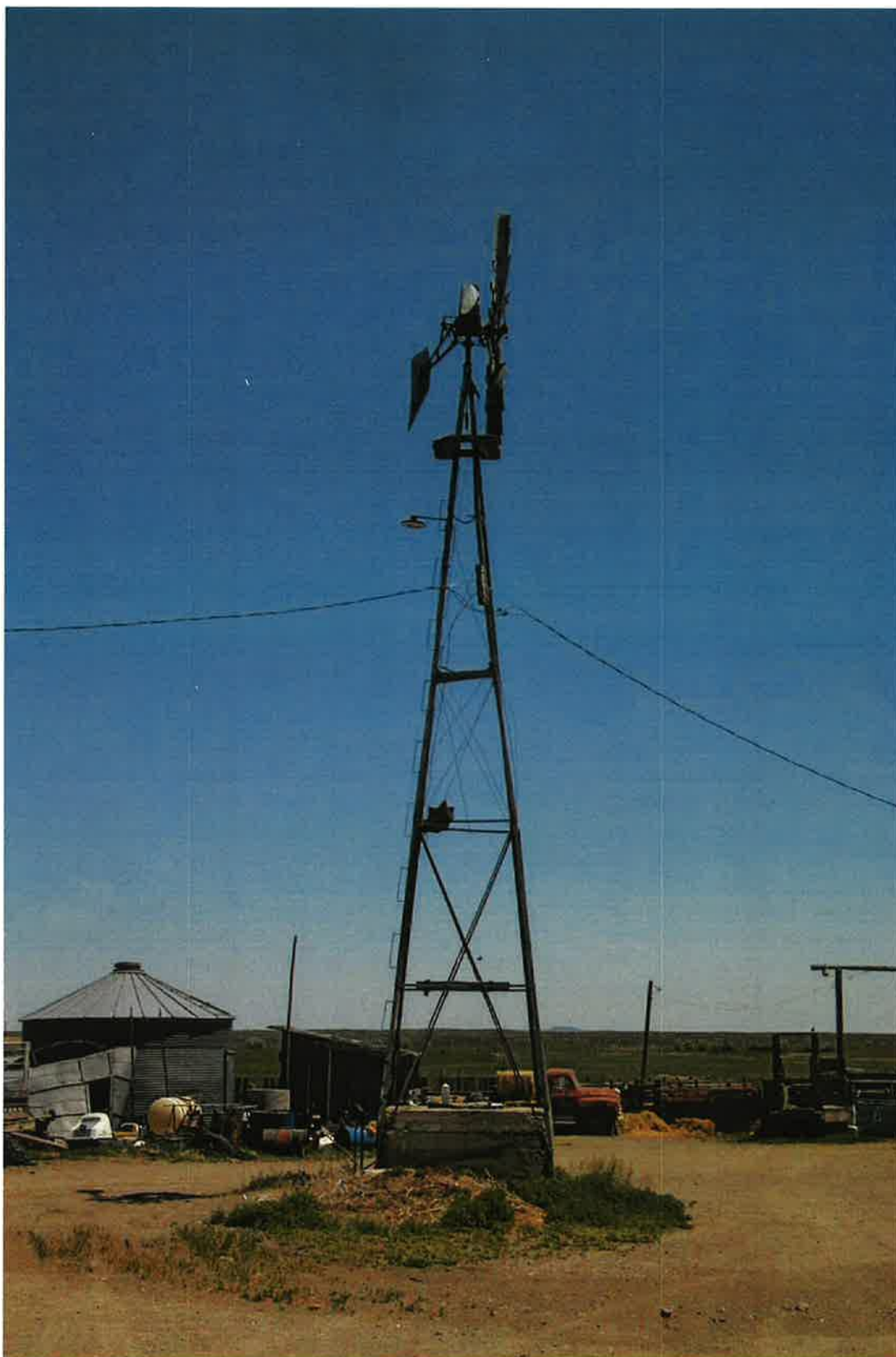
Well is at the base of the windmill. Submersible electric pump is set at the bottom of the well. CLF 5-31-02
