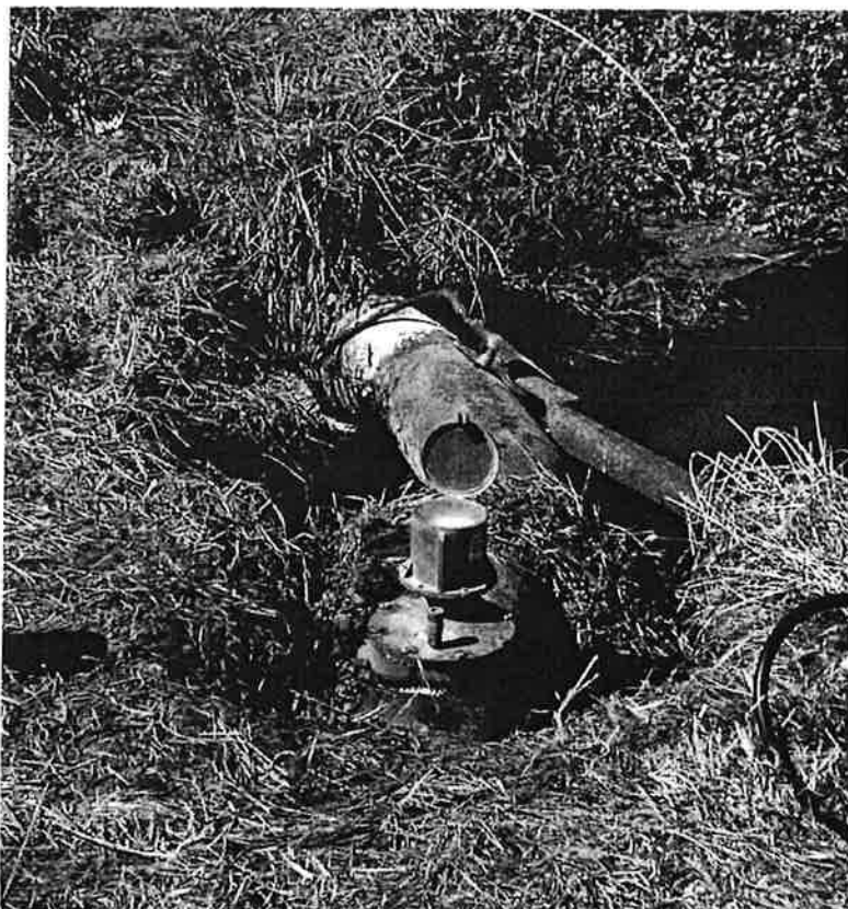
Gravity irrigation flowmeter, located just outside powerhouse
