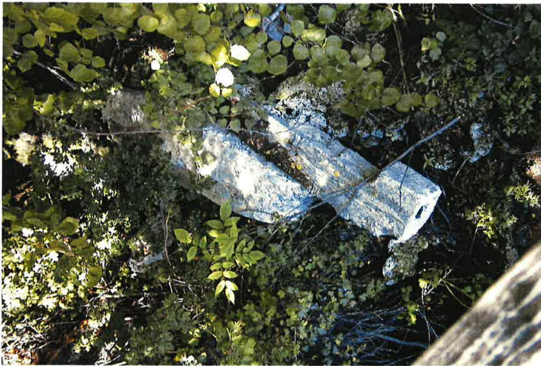
Remains of old power plant structure
