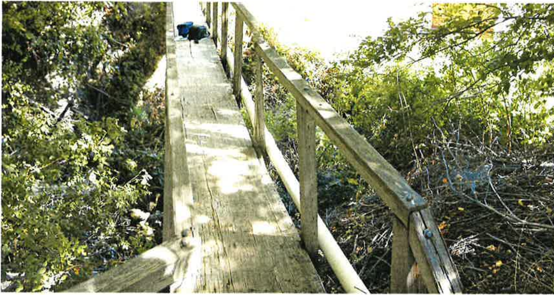
Bridge over stream to power plant. (Remains of original structure was below on left.)
