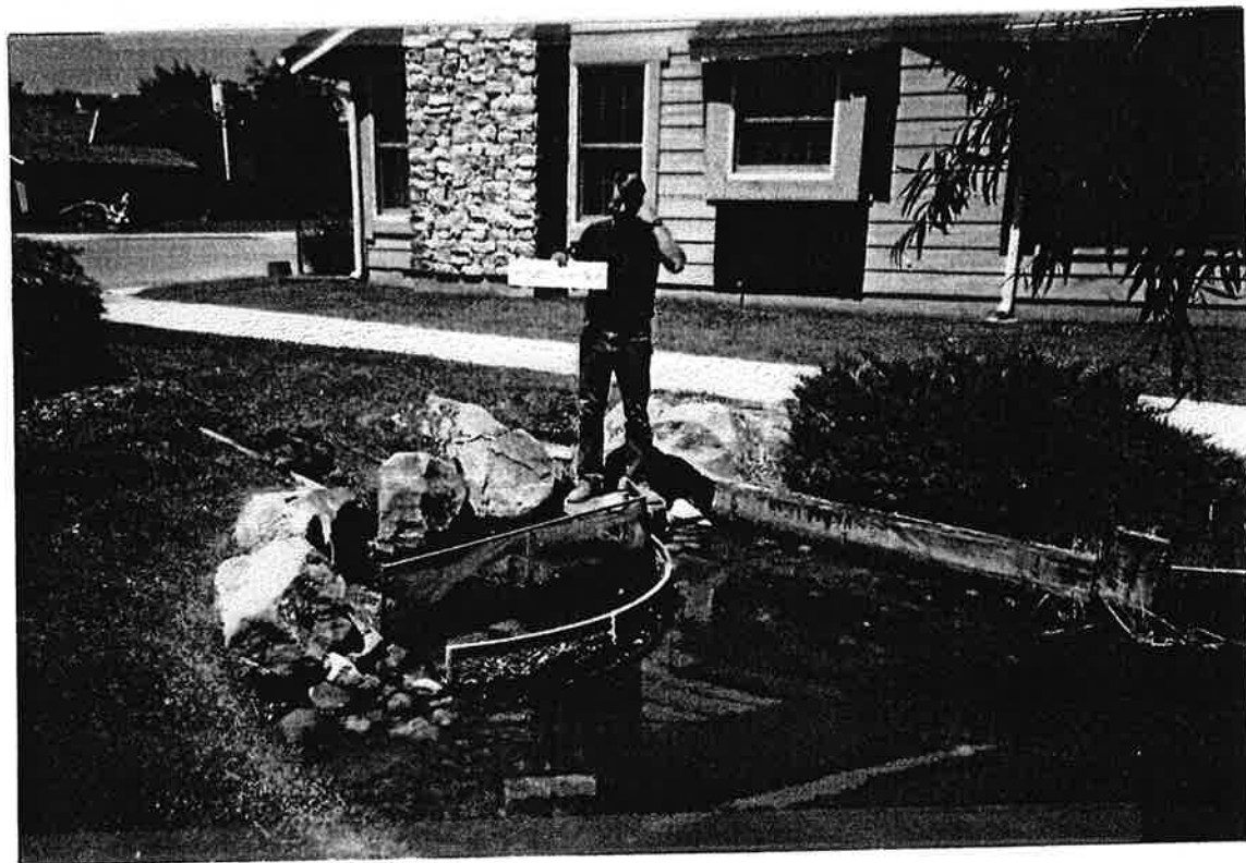
Point 12 Adjacent to Pump House Permit 63-08402 on Raindrop Drive.
