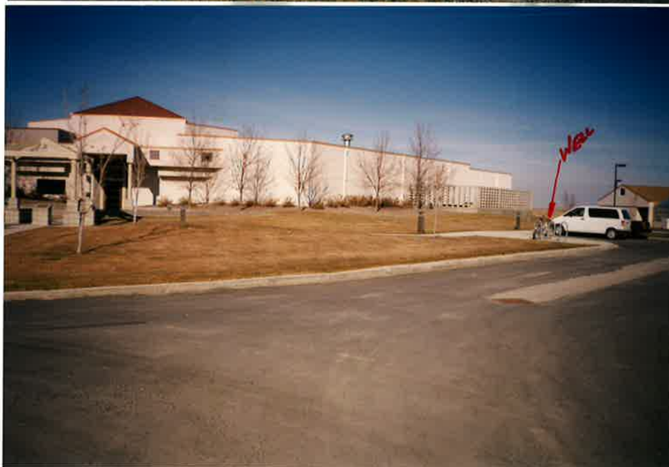
Photo 3. Front of Main Research Facility Building Looking North. Compares to Photo 4 Right Hand Side.
