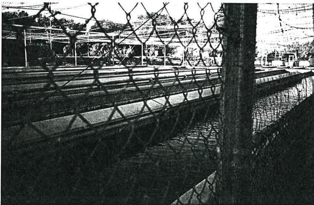
* SHOWS RACEWAYS - FACES SOUTHWEST
