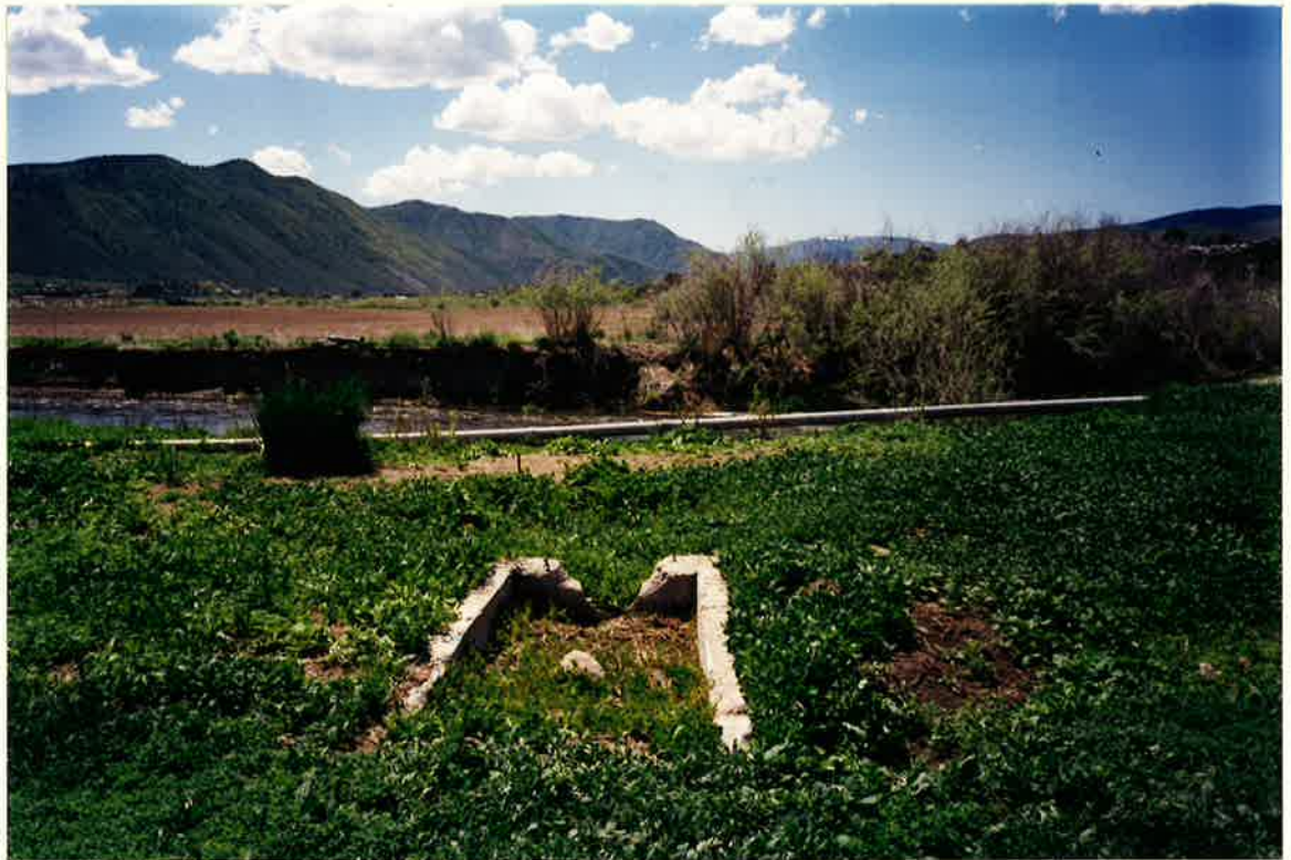
Looking West at Concrete structure used to Hold historical Pump. Portneuf River in Picture.
