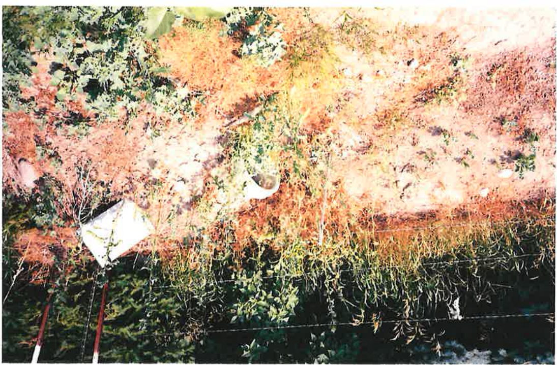
Looking N. Culvert that delivers water from ditch to cleared POU.
