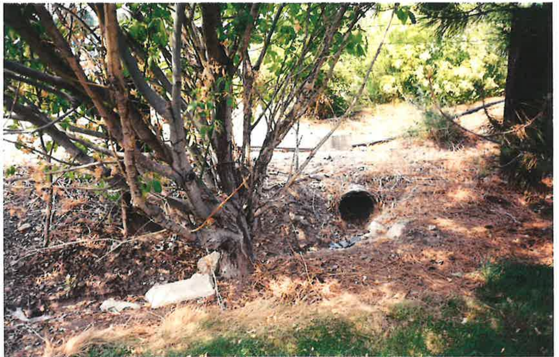
Culvert that leads to Chavers place
