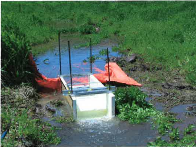
Photo 1. Installed Broad-Crested Weir.
