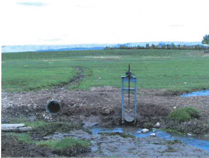
Photo 1. Wilder's diversion ditch on the right.
