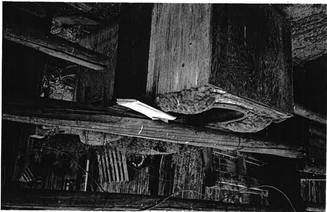
Looking @ what is assumed to house Eastern most well
