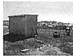
PUMP HOUSE AND POINT OF DIVERSION 1
