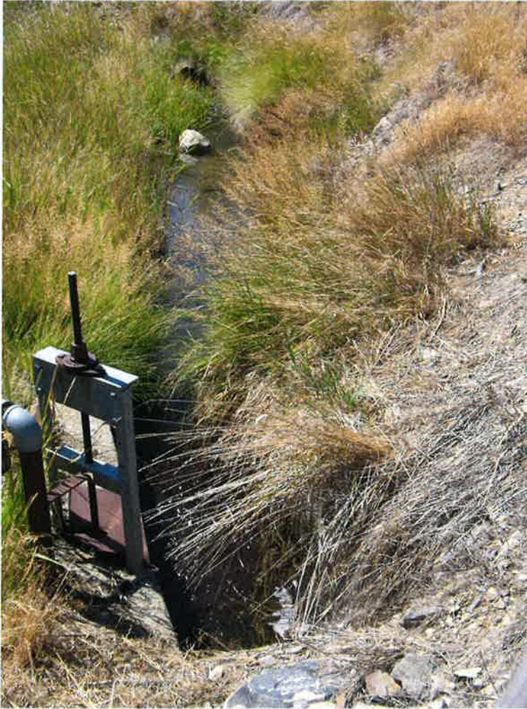
Alternative view of the headgate in the previous picture. Upstream is to the front of the viewer and downstream is to the left.
