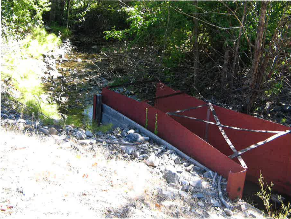
This photo was taken standing at the Farmers Ditch headgate and looking downstream along Farmers Ditch. This picture was taken facing north. The confluence of Jesse Creek and Pollard (Canyon) Creek is just behind the picture taker.
