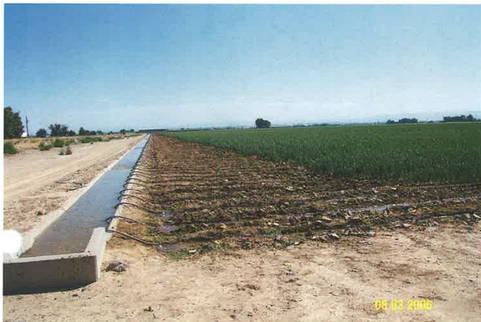
EAST FIELD LOOKING SOUTH
