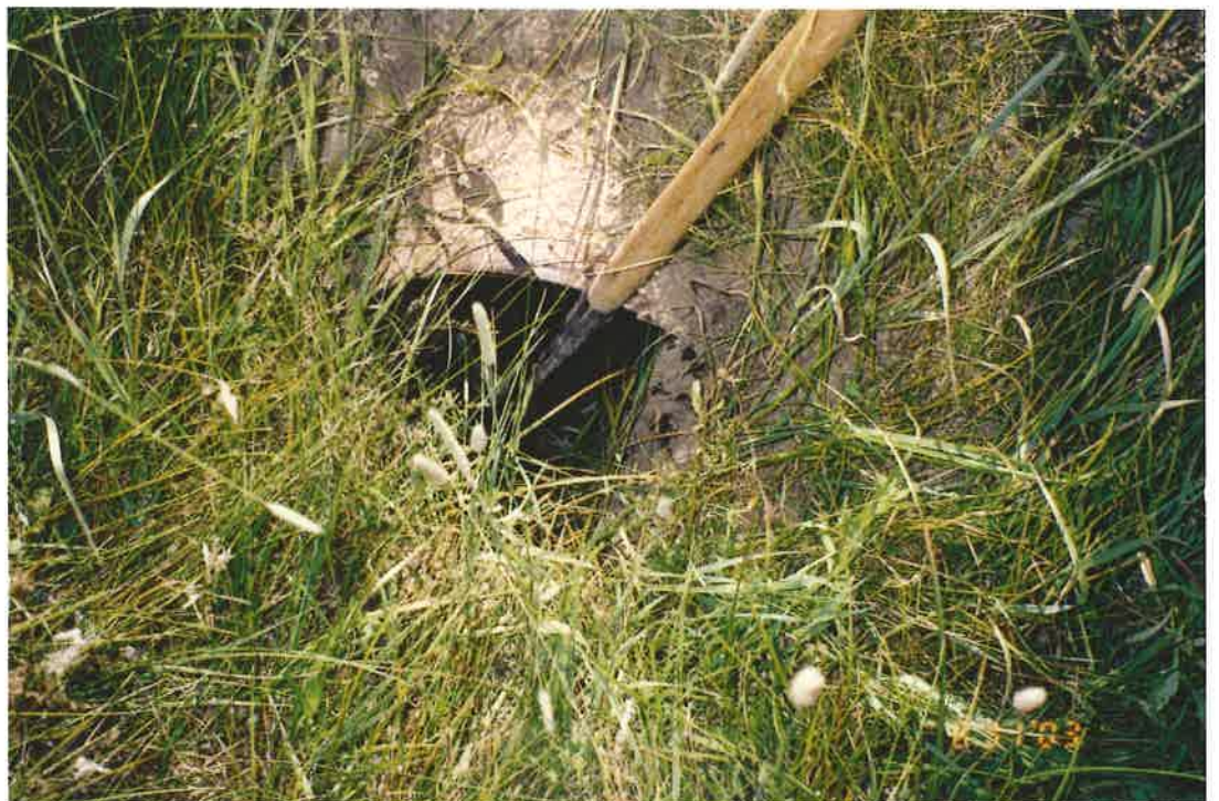
Upper Culvert in NENE S11
