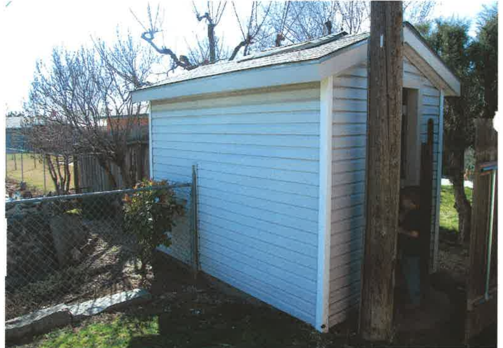
Pump House Looking Southwest
