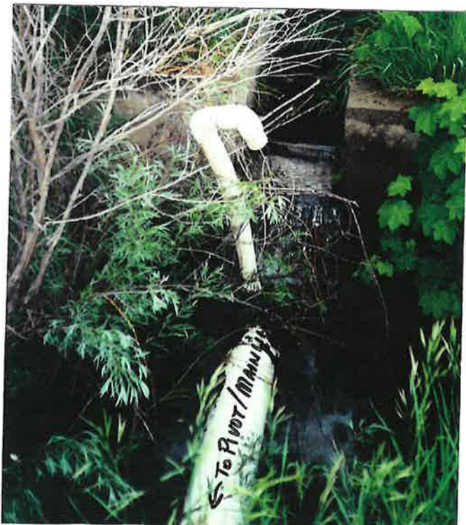
← Photo 3: SHOWS INLET TO MAIN- LINE GOING TO PIVOT
