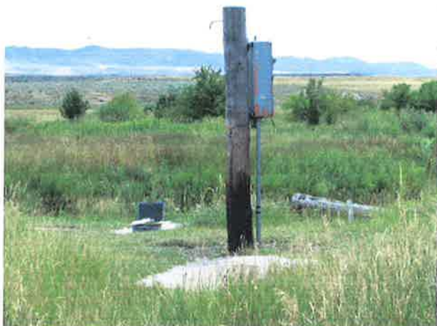
Photo 1. Diversion point from Marsh Creek.
