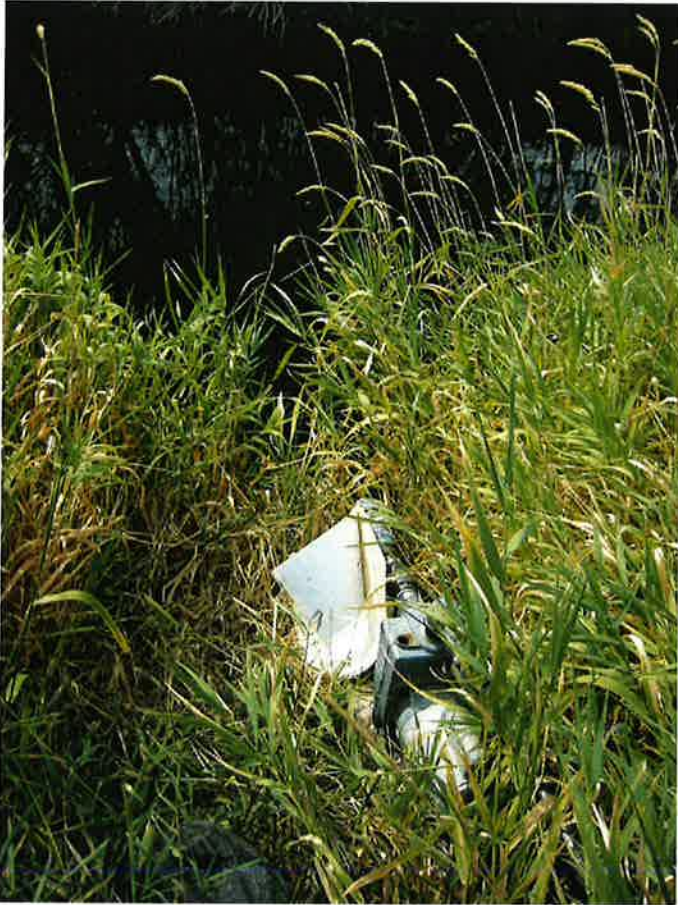
Looking South at pump. Portneuf river at the top of picture. POU behind me in Picture.
