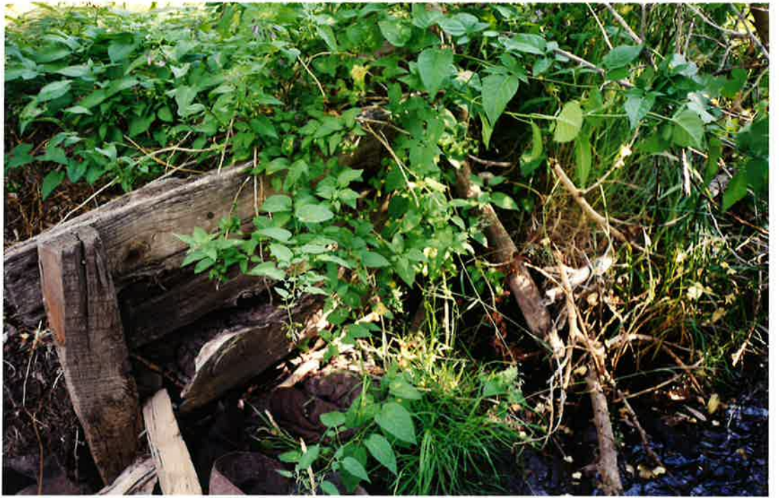
Headgate used to divert Rapid Cr water
