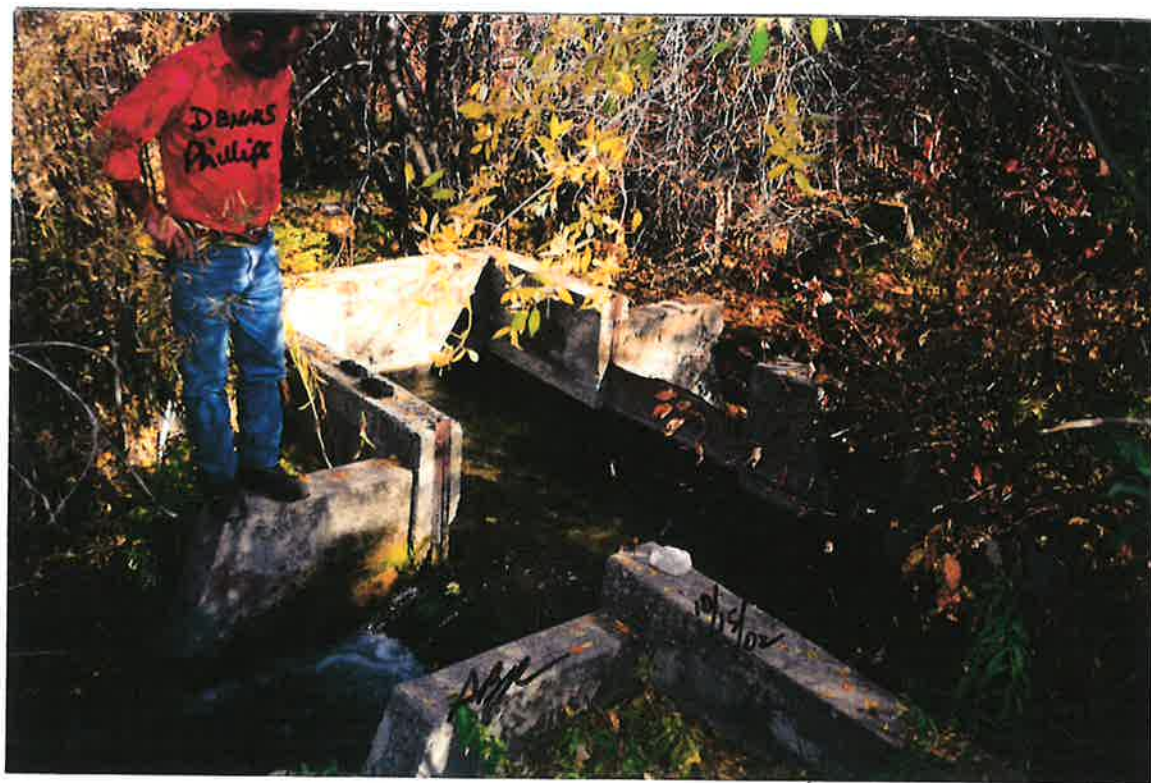
RB-DW. Sec. 23 125/365 LOWER DIVERSION (JUST OFF IIS: E. SIDE) DIVIDES BIRCH CK (ON MARSH CK SIDE). DENNIS PHILLIPS, WATERMASTER, STANDS AT THE SIDE THAT GOES ON TO NW, PIPED UNDER IIS TO BIRCH CK CANAL.
