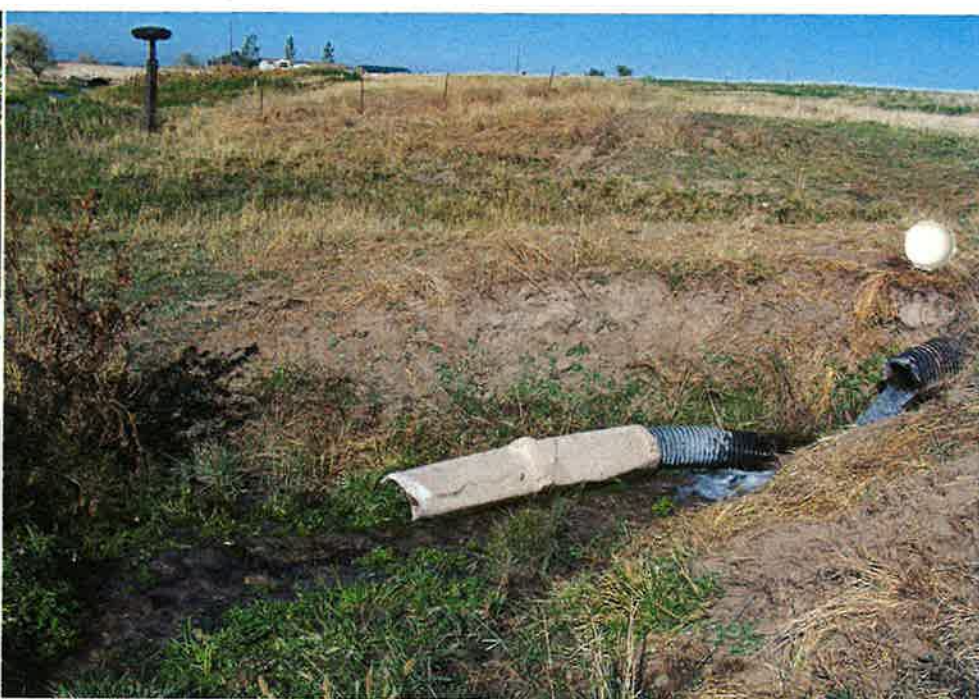
↳ over flow to 12" buried pipe to creek →
