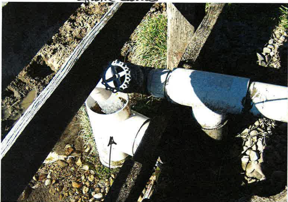
↳ over flow to 12" buried pipe to creek →
