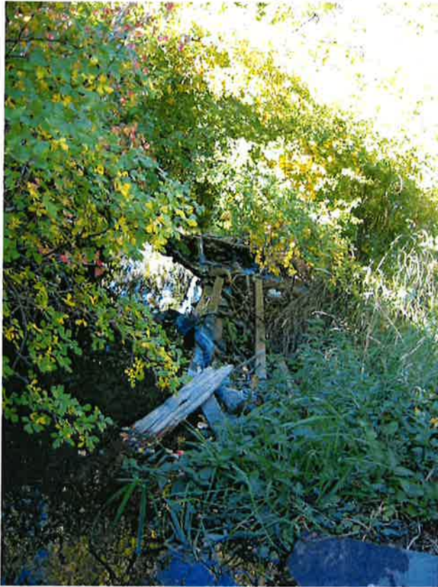
Looking West at POD where water is diverted from the main channel of Mink Ck to ditch system.
