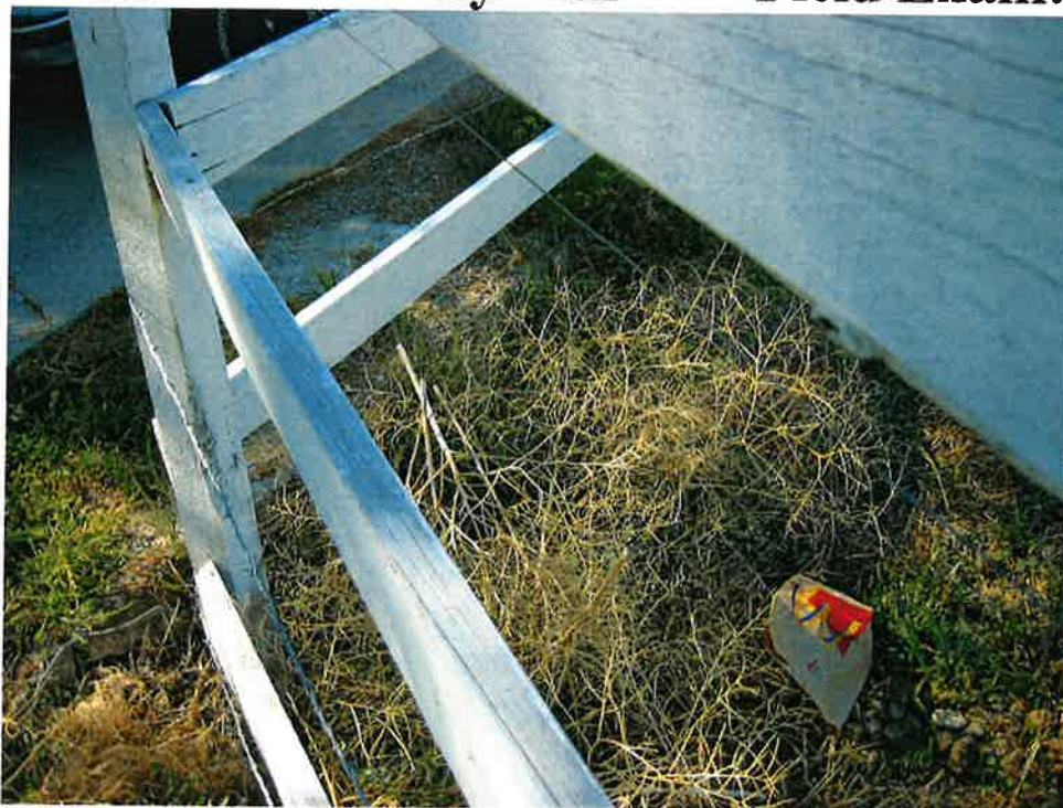
Looking at what is a now filled in culvert that carried water from Mink creek to the claimed POU.
