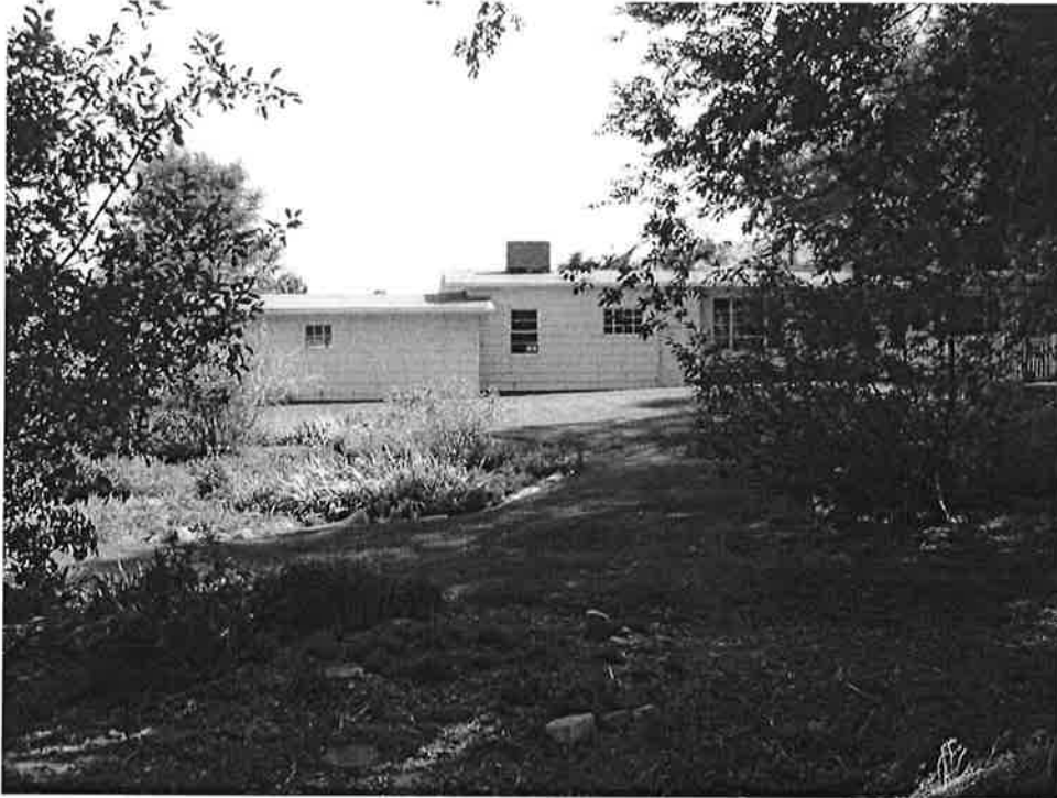
Looking S at claimed POU. Back yard. House in background of picture.
