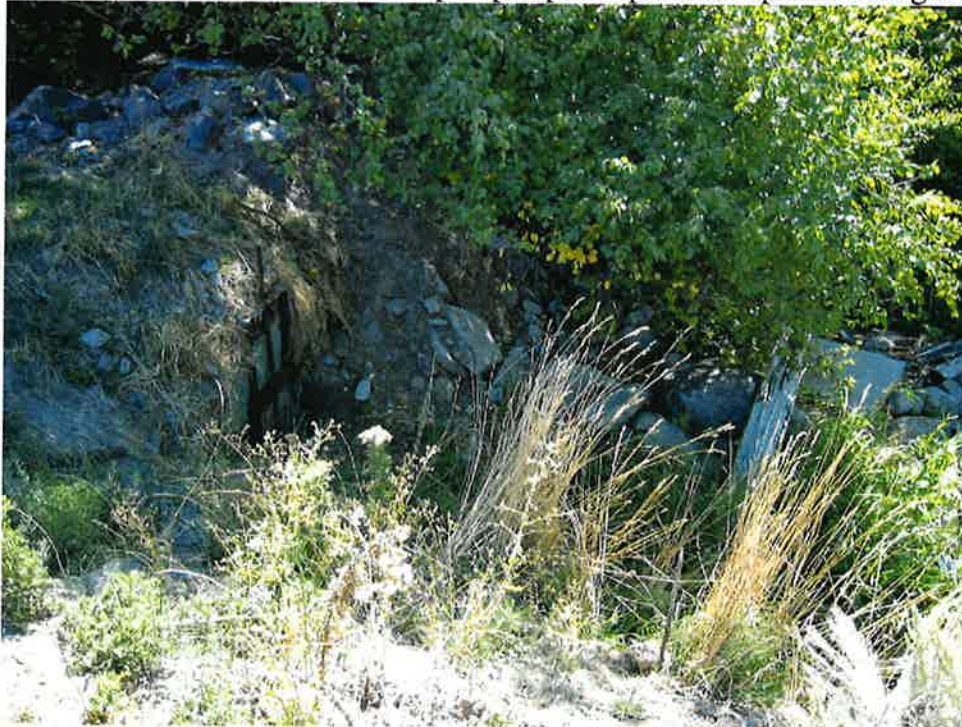
Looking West at head gate that is opened to supply water to flood irrigation ditch. Mink creek (to the right of the picture) would have to be pretty high to get water to the head gate.
