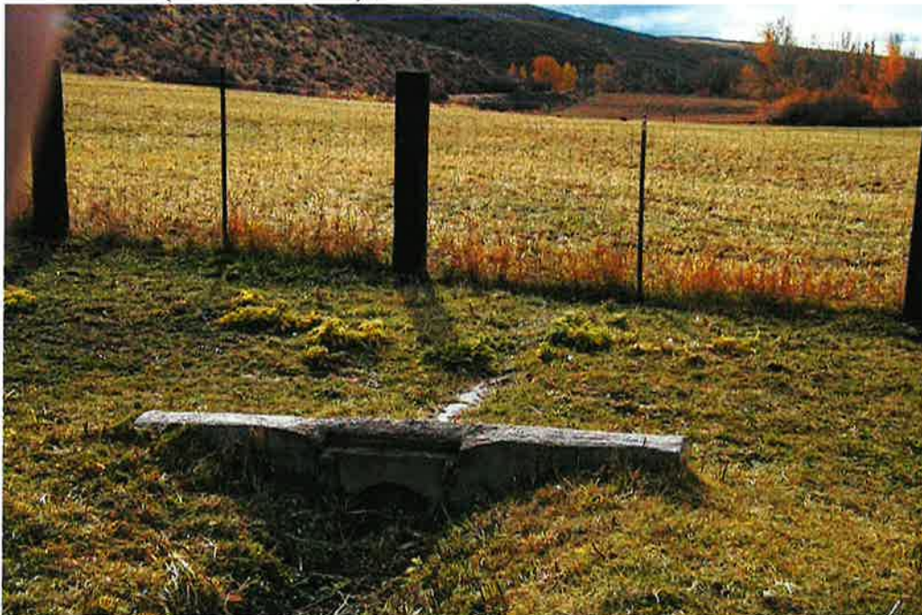
Looking South. South end of claimants property. Sam Chandlers property in the background. Culvert that conveys water to Sam's property (csaxton 11/02/01).
