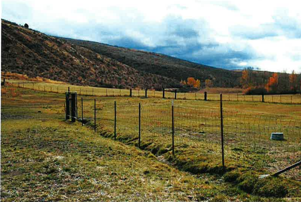
Looking South. Portion of original ditch that was not covered by the claimant. POU to East and West of ditch (csaxton 11/02/01).
