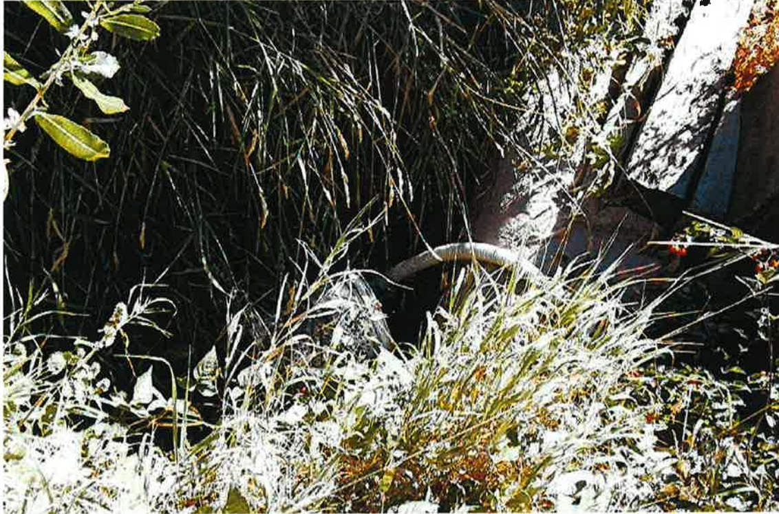
Intake line for pump drops into Pocatello Creek. POU and pump behind me in picture. (csaxton 10/8/01).
