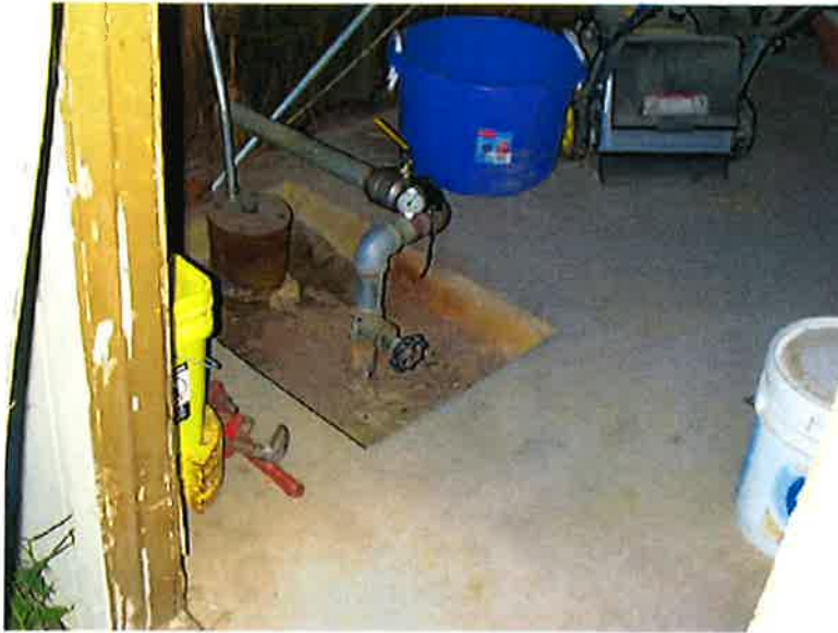
Facing SW looking into pump house.
